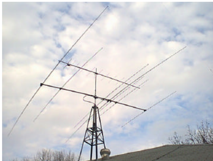
K2CS Beam. Force 12 C3 on a 9-foot Glen Martin rooftop tower. Nothing fancy or tall, but it beats a wire on the high bands.
