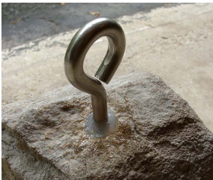
Screw eye installed and sealed against moisture penetration.
