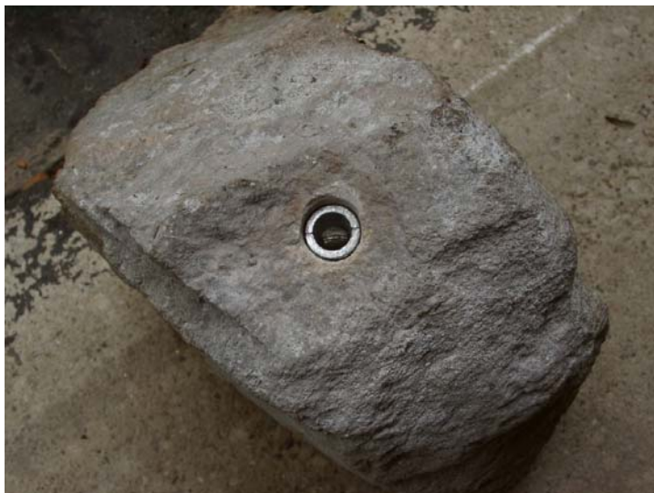
Completed mounting hole with lag shield inserted. Hole is slightly deeper than the length of the shield; permits complete sealing of hole with silicone.
