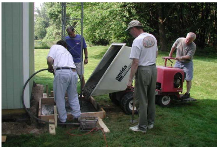
The “power buggy” and concrete pour.
