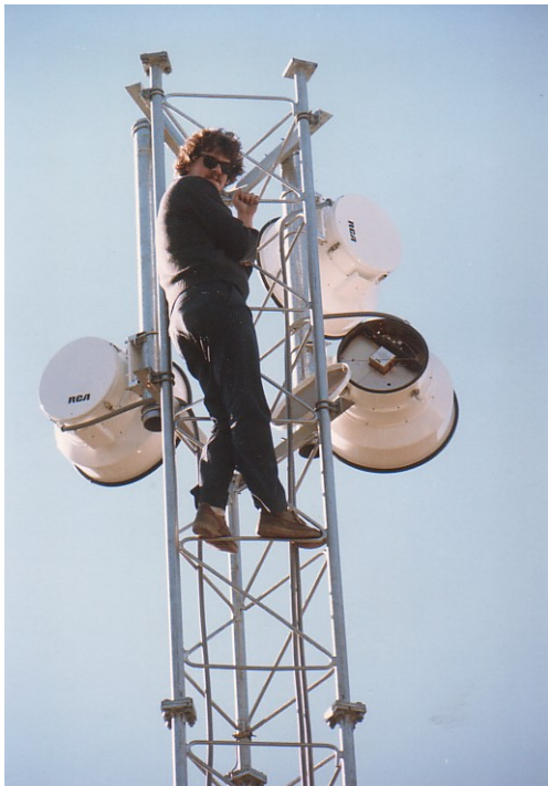
Chris, K2CS: in the early 80s at the Miller Brewing Company, Baldwinsville (Syracuse) NY. The dishes are 10GHz and were built by RCA to transmit line of site video signals to cameras around the brewery. Ironically enough, I spied these dishes many years later at one of the hamfests I attended, as they made their way into the ham radio VHF world.
