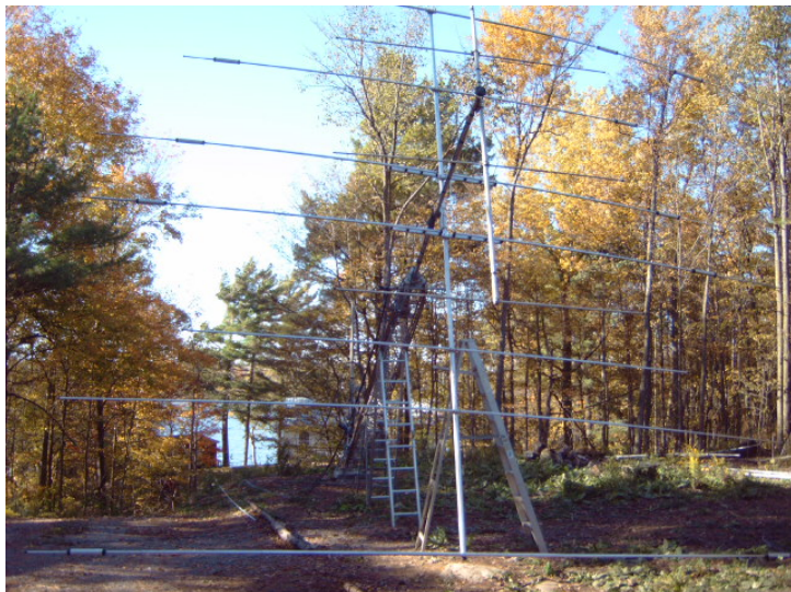
Mosley Pro 67B fully assembled and mounted on the tower prior to raising.
