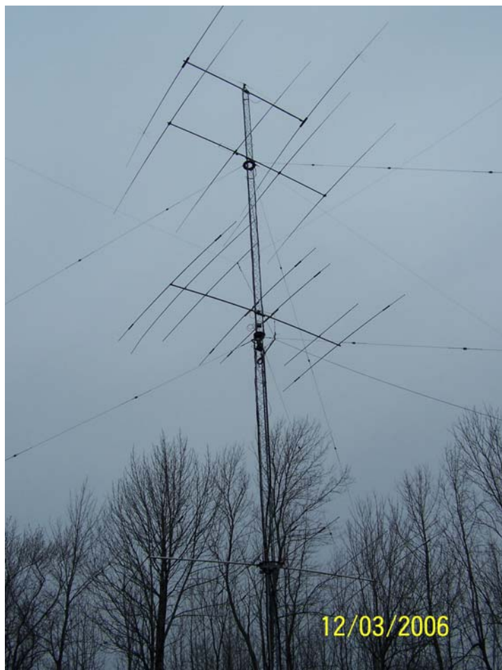
Tower #1 Rohn 25G , 110 feet, top 50 feet rotates. 2 el 40m Cushcraft @ 109 ft.; 4el 20m Hygain @ 92 ft.; 2, Mosley Pro 57As @ 62 ft. and 32 ft., stacked using Array Solution stack match unit. The tower also supports a 160m sloper.
