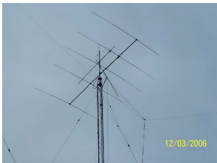
Tower #2 Rohn 25G foldover , 68 feet. Cushcraft ringo at top; 5 el 15m Hygain @ 70 ft.; 14 el 2m Cushcraft @ 78 ft. The tower also supports an 80m horizontal loop.
