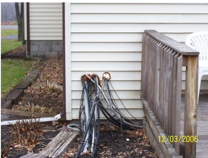
What goes up must come in. An outside view of the feed and control line entry point.
