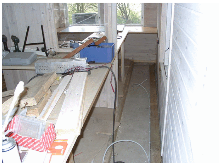
Passage way behind operating positions for rear panel access. The equipment room is behind the wall to the right. The wide gray strip seen on the floor, running parallel to the operating desks, is actually a cable duct, with a pass-through under the wall into the equipment room. Removable flooring will cover the duct once cables are in place.
