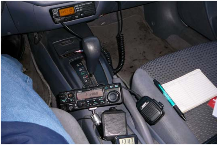
The finished installation.
