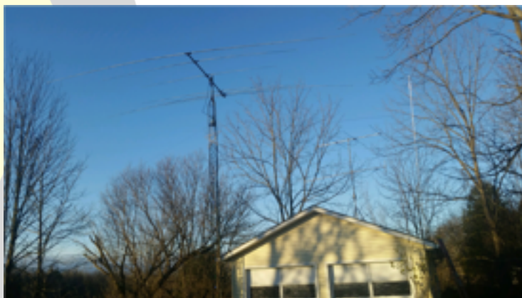
Antenna farm in daylight, rebuilt C3S, HF9V on right, VHF stack in the middle (Hygain VB-64, Cushcraft 13B2)
