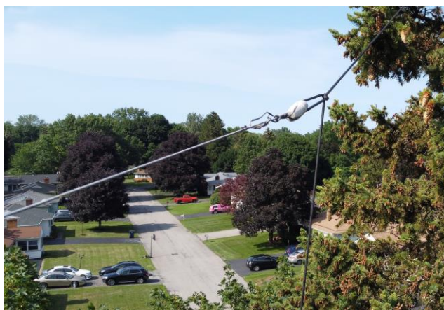
160m inverted-L end insulator at 60 feet
